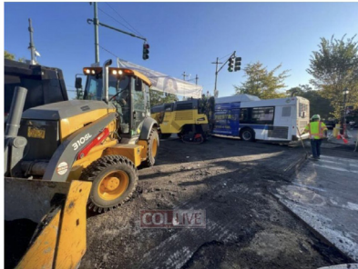
Provided regular community updates regarding issues affecting the community
