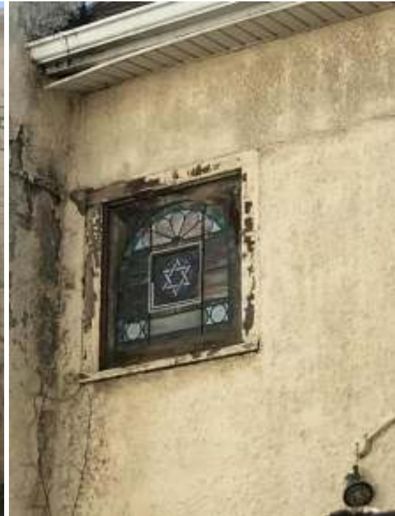
Rear of building, window detail
