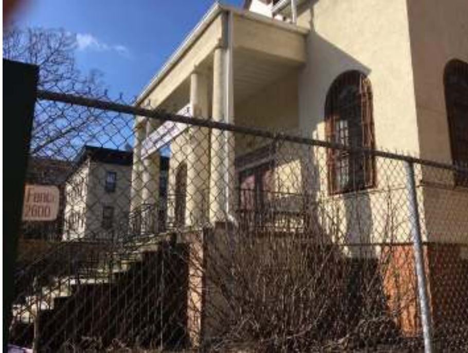
Porch: side view
